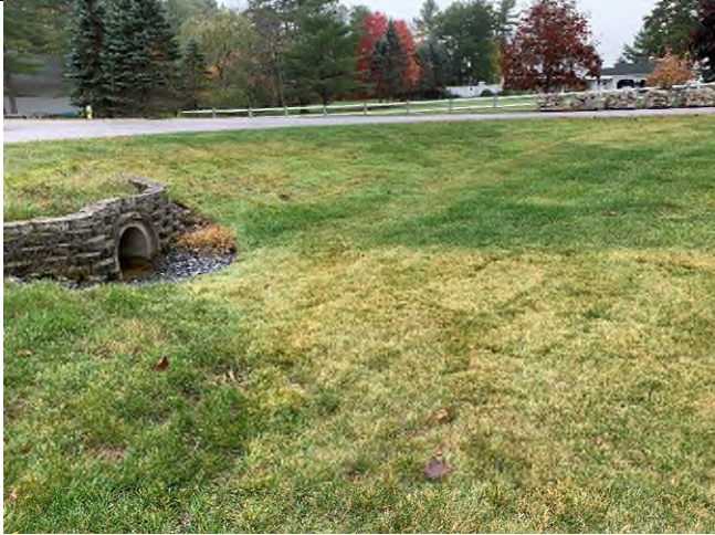
29 Gundalow - 1 (Drainage Area)
