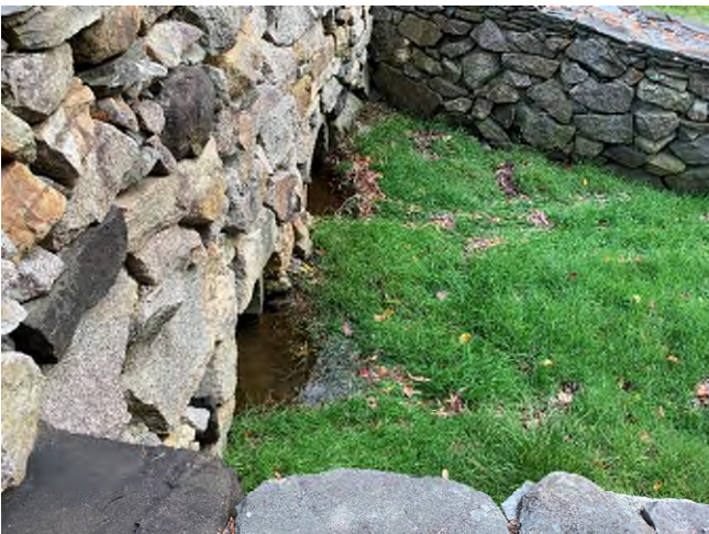
4 Brickyard Circle - 1 (Drainage Course)
