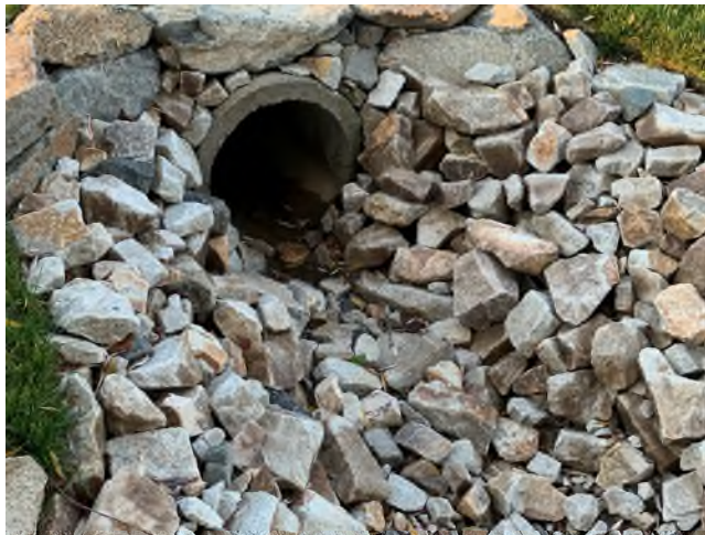
64 Gundalow - 1 (Drainage Course)
