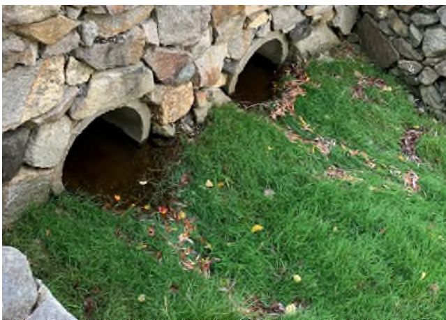
4 Brickyard Circle - 1 (Drainage Course)
