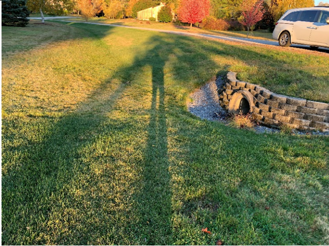
29 Gundalow -1 (Drainage Area)
