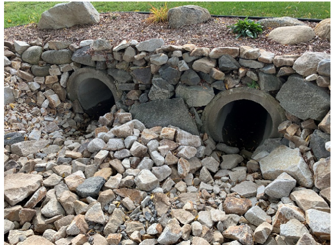
64 Gundalow - 2 (Drainage Course)
