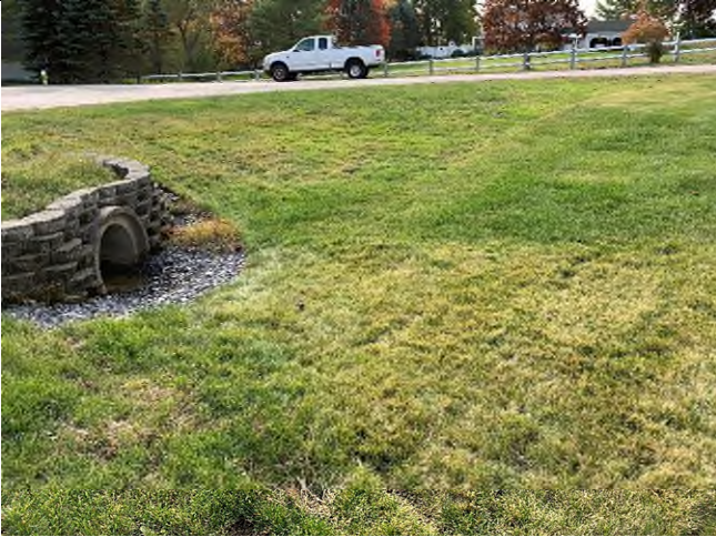
29 Gundalow - 1 (Drainage Area)
