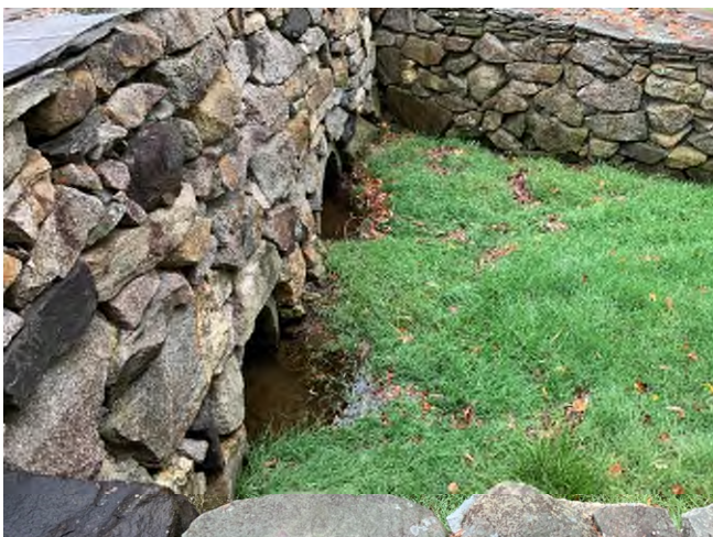
4 Brickyard Circle - 1 (Drainage Course)
