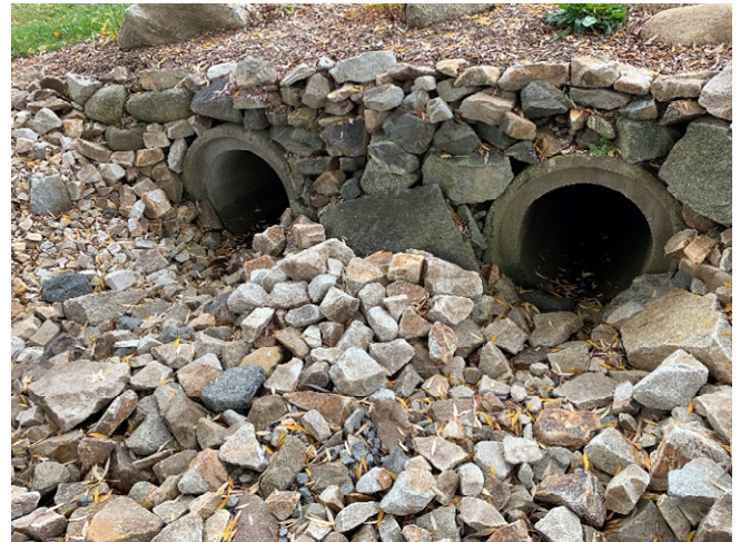
64 Gundalow - 2 (Drainage Course)
