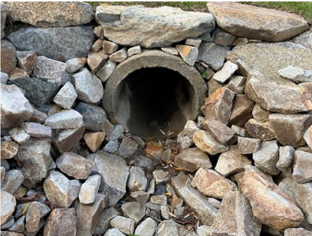
64 Gundalow - 1 (Drainage Course)
