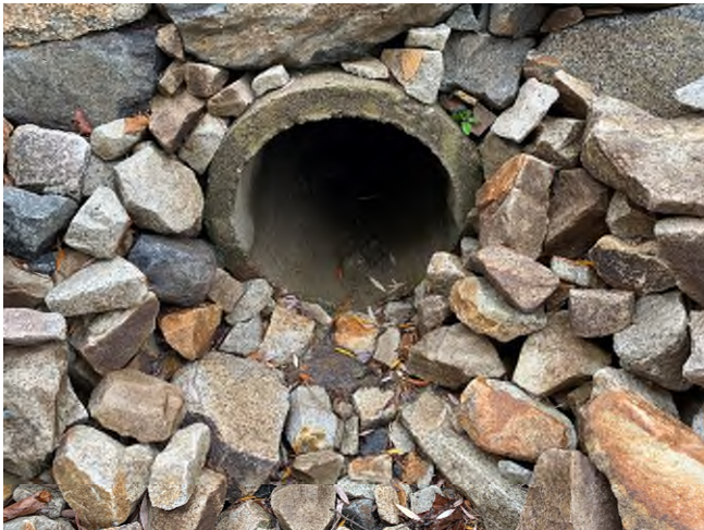
64 Gundalow - 1 (Drainage Course)
