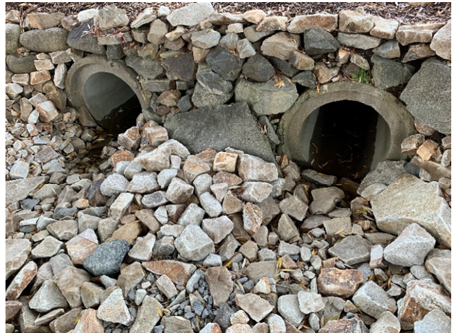
64 Gundalow - 2 (Drainage Course)
